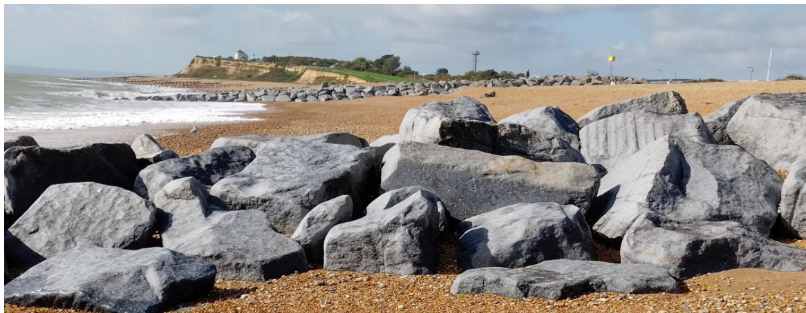
Rocks on the beach at Glyne Gap to prevent erosion; Galley Hill in the distance to the west
